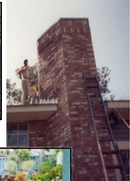
Trojan being sprayed on masonry
