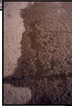
Before and After concrete repair on sidewalk using Bondex 201
