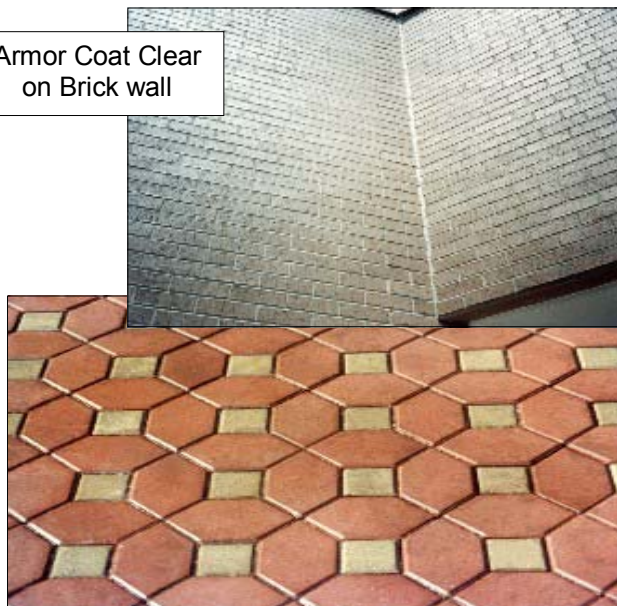
Brick Pavers Sealed with Armor Coat Clear Finish
