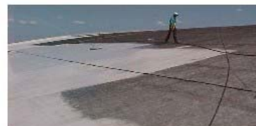
Roof Cleaning at Panther Stadium, Sunrise, Florida (The grey areas are mildewed The white areas have been cleaned)
